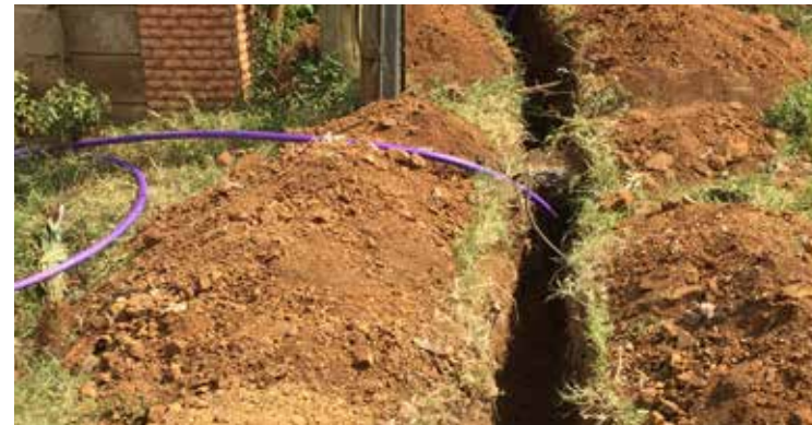
Liquid Telecom Kenya lays cable 1.2 meters deep
